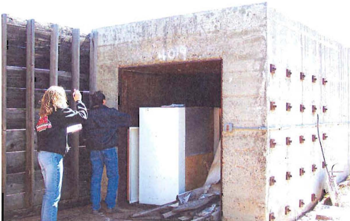
TA-6-9, Northeast wall and northwest wall of southern portion of building, direction south
