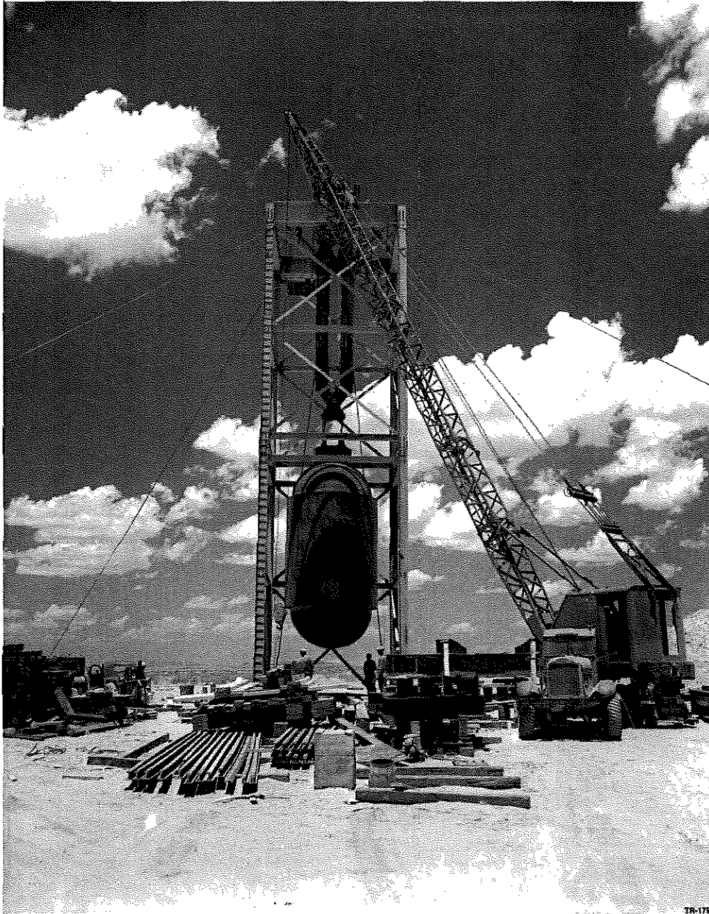
Figure 19. Jumbo on Tower Structure at Trinity Site, 1945
