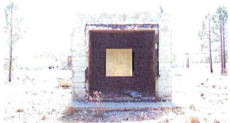
TA-6-7, Northwest Elevation, April 2004 (after Cerro Grande Fire)
