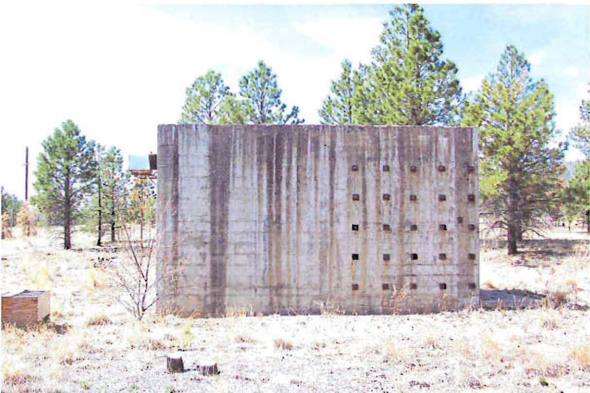
TA-6-7, Northeast Elevation
