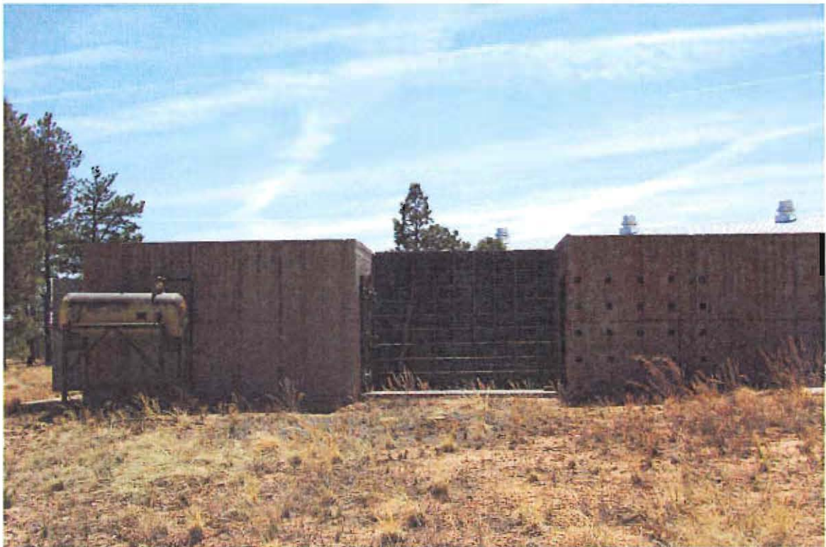
TA-6-9, Northwest Elevation
