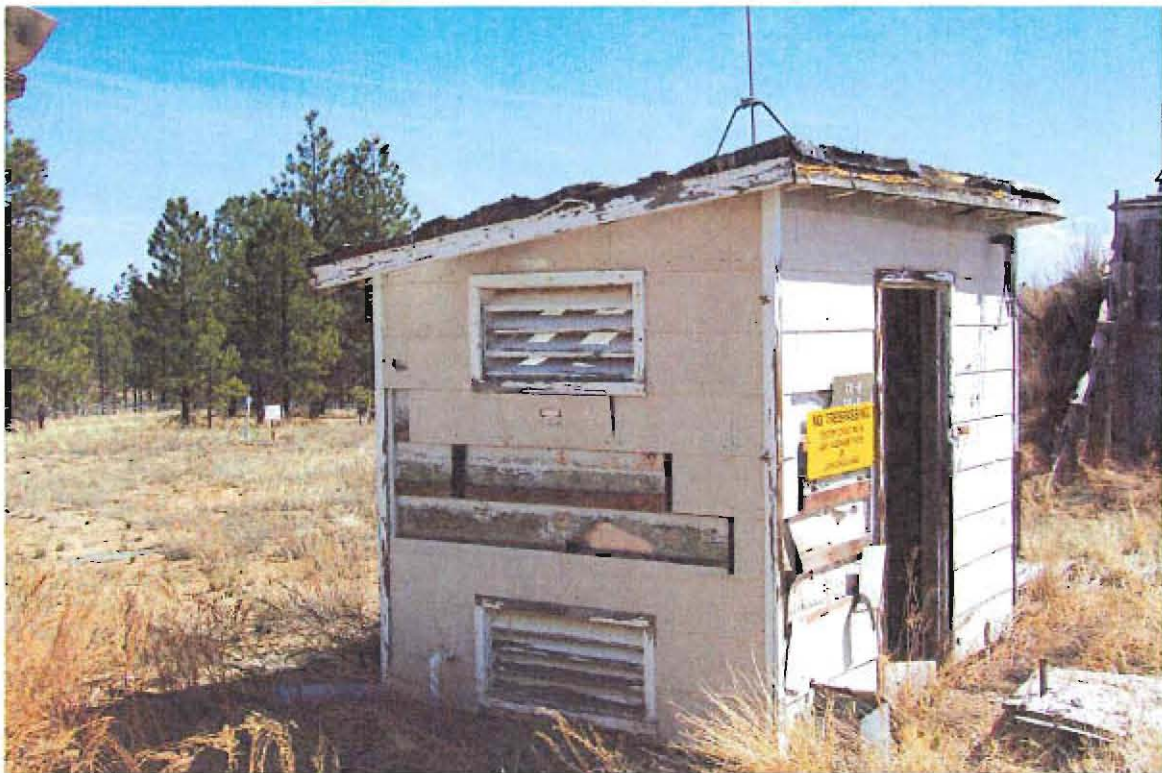
TA-6-2, West and South Elevations
