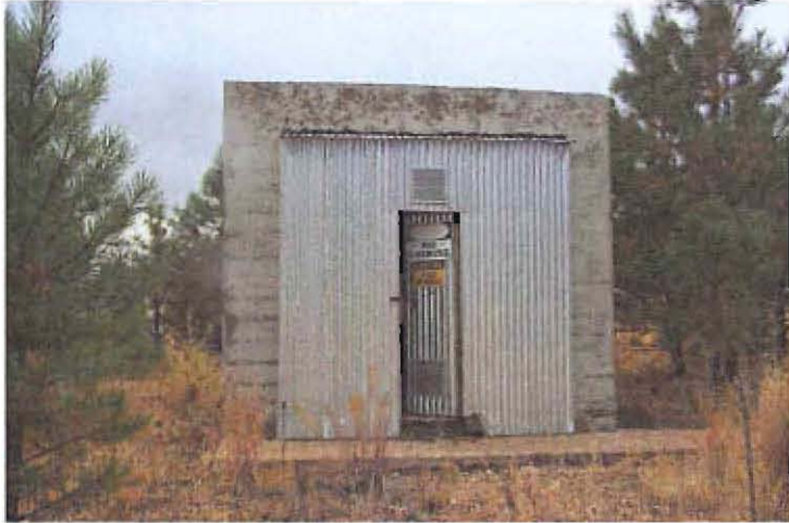
TA-6-7, Northwest Elevation, October 1999
